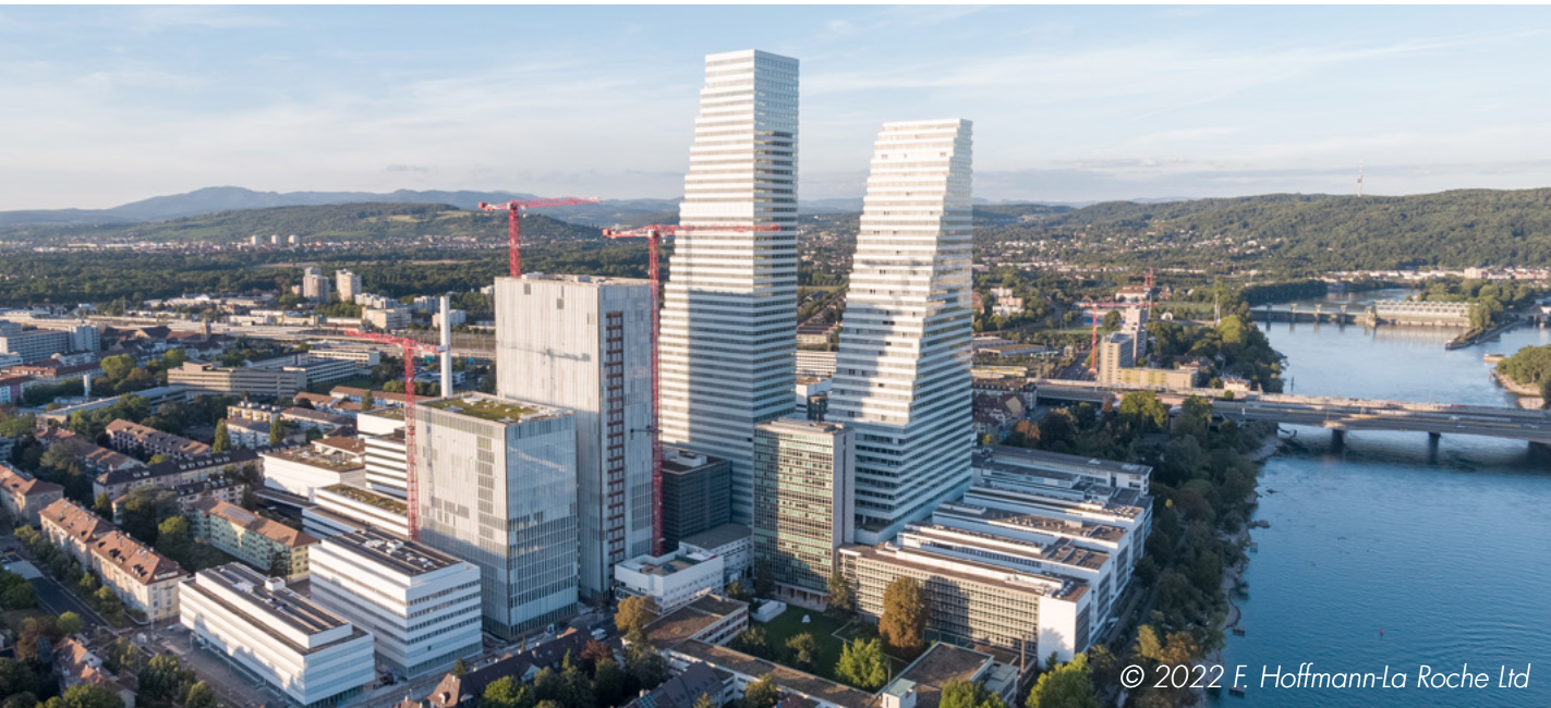
The two iconic buildings on the Roche premises in the Wettstein district of Basel.
