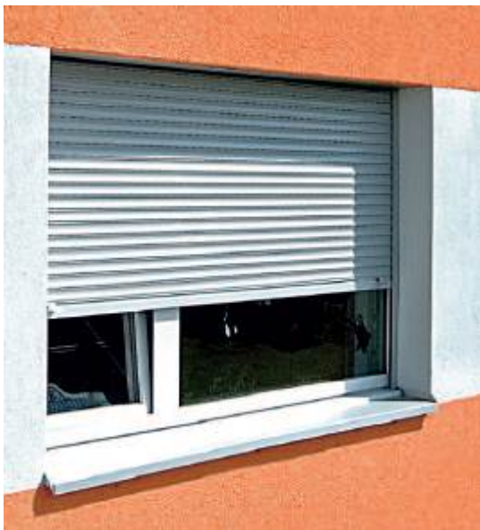
Fig. 3: Built-in roller shutter (Source: Griesser brochure on roller shutters)
